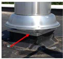
Exhaust fan with no base fasteners
