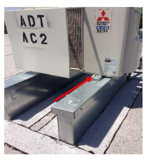
Split HVAC unit not secured to its curb
