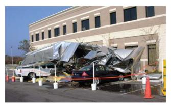
Even larger, heavier equipment may be blown off the roof when securement is deficient.
