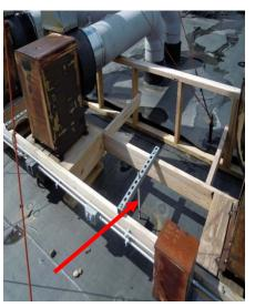
Sleeper mounted equipment secured with iron rods via pitch pockets
