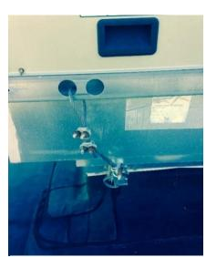
Packaged HVAC unit secured to curb using angle iron & cable ties
