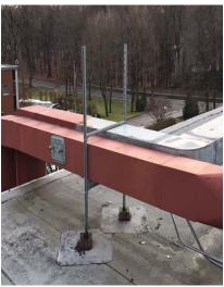
Ductwork secured using brackets via pitch pockets
