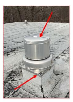
Well secured curb mounted exhaust fan; use two straps in high wind zones
