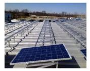
While mechanically secured, this system lacks fasteners at every seam
